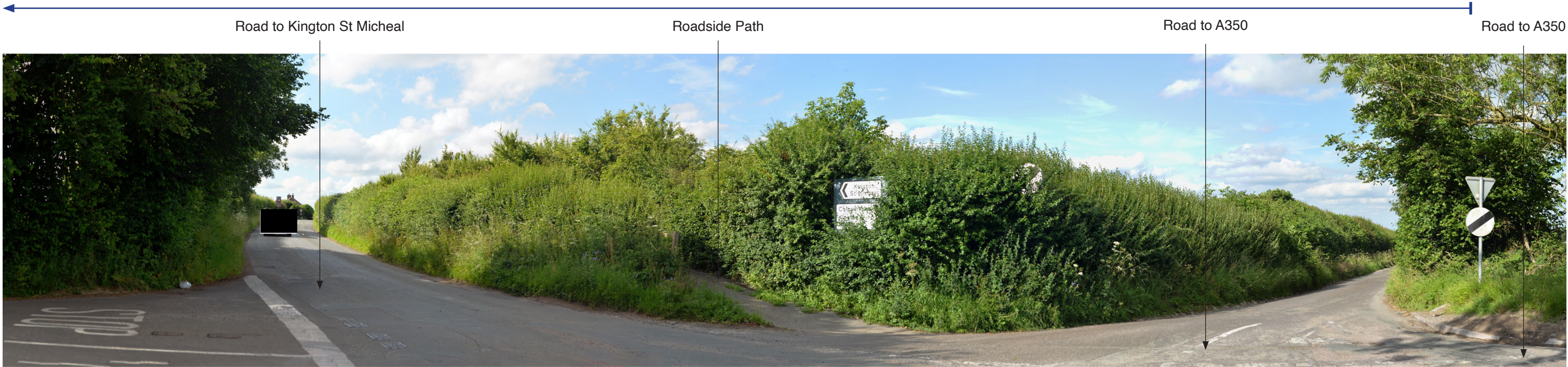
ASVP 10: From road junction looking north
